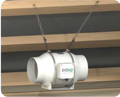
Suspend the fan with chain
